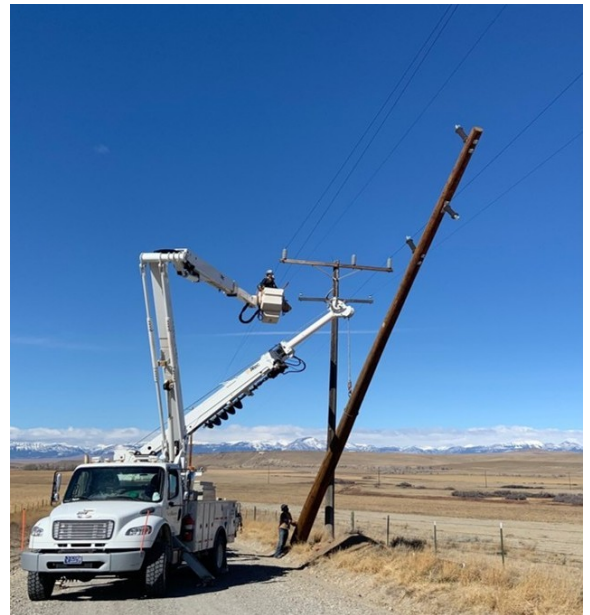
A NorthWestern Energy crew replaces a power pole dangerous to birds with a new pole that is avian safe.
